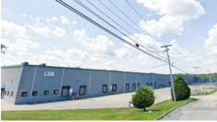
The building in question stretches 1,600 feet down and was a lot of area to cover for Norwood Firefighters.
