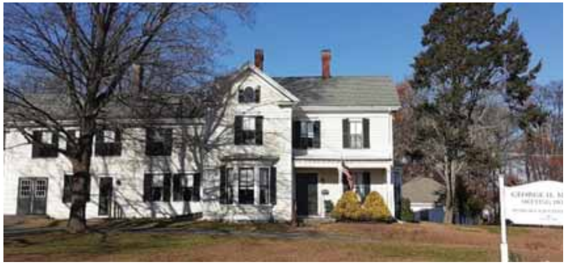
The George Morse House in Norwood has been standing for at least 100 years and residents are advocating for its renovation.
