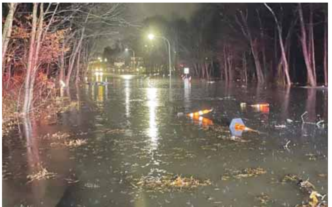
The flooding at Upland Road/Route 1A in January was found to potentially have been caused by a clogged storm drain.
