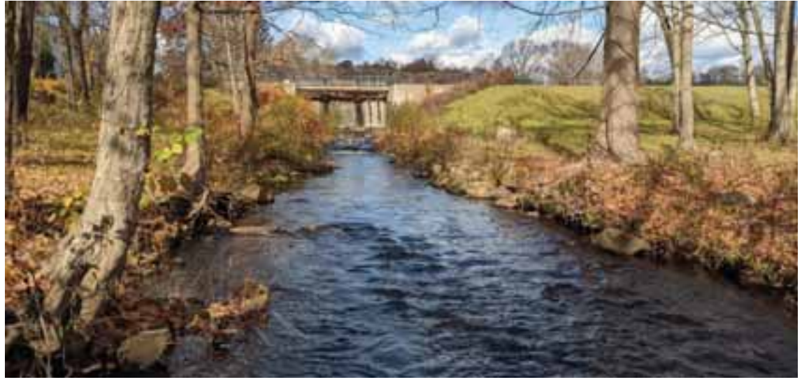
The ConCom approved dam work on the Ellis Pond Dam that will hopefully keep the machinery in working order for years to come.
