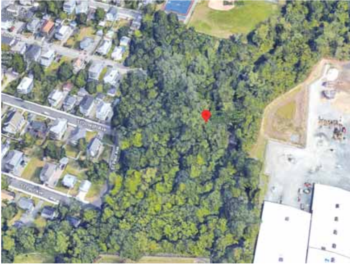
Construction has started at the Bernie Cooper Memorial Riverfront Park in South Norwood.
