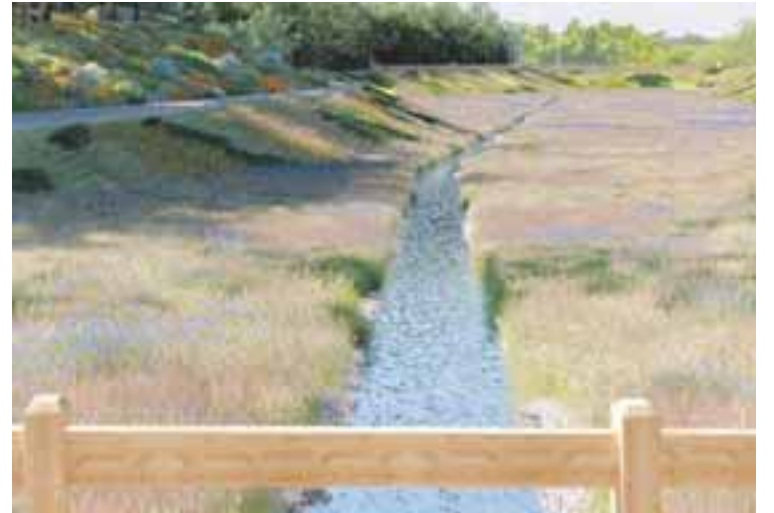
The Norwood Ad Hoc Stormwater Committee discussed how to sell the Town on the Hennessey Field Drainage Basin project.
