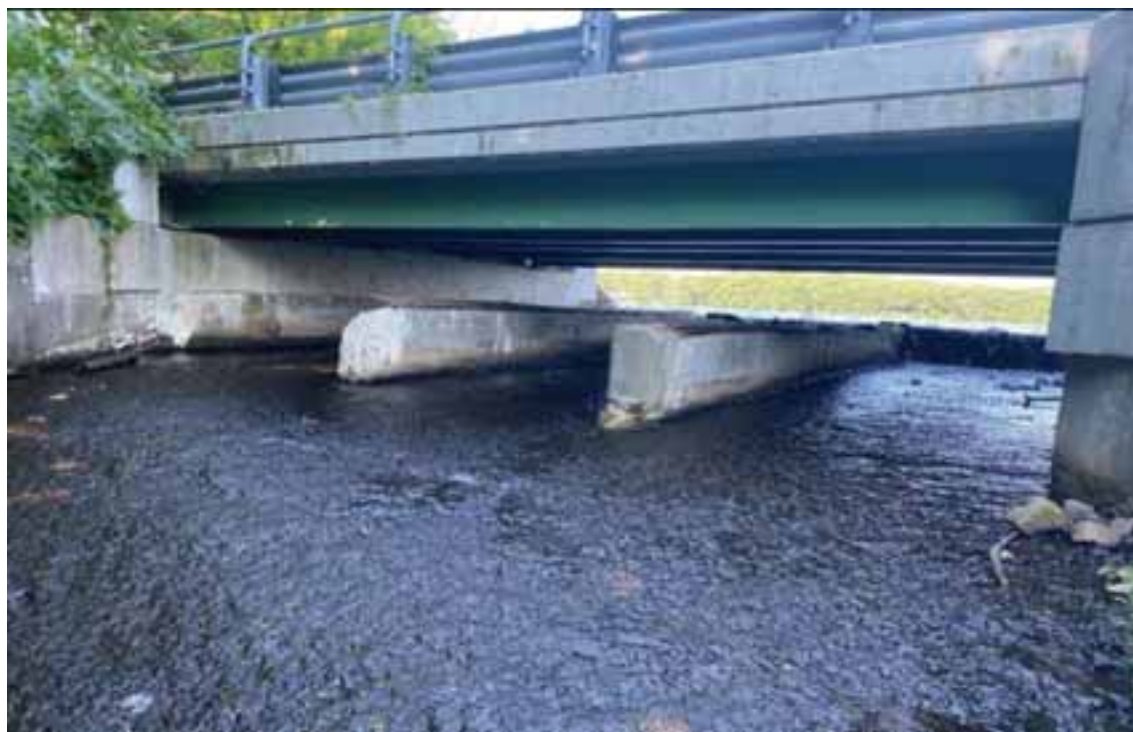
The repairs include replacing a trash-catching device to make sure debris doesn't interfere with the operation of the spillway.
