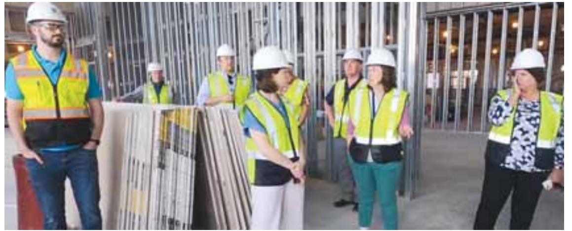
Norwood Public Schools staff and the Middle School Building Committee took a tour of the Coakley Middle School construction site recently.
