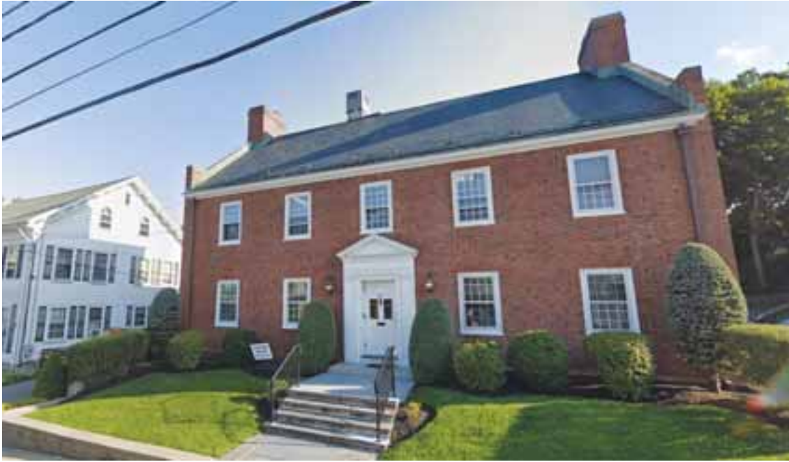
The current site at 20 Vernon St., which is slated for veterans housing if the proposal goes through Town Meeting.
