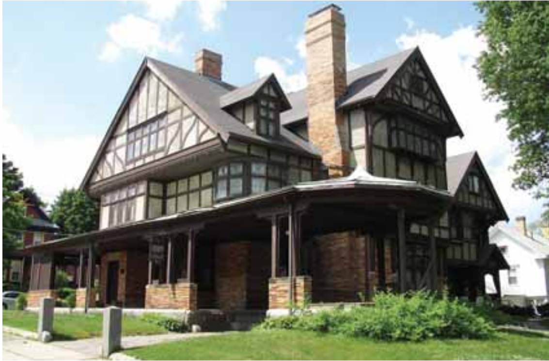
The Day House in Norwood will see improvements if Town Meeting approves the funding application to the Community Preservation Committee.
