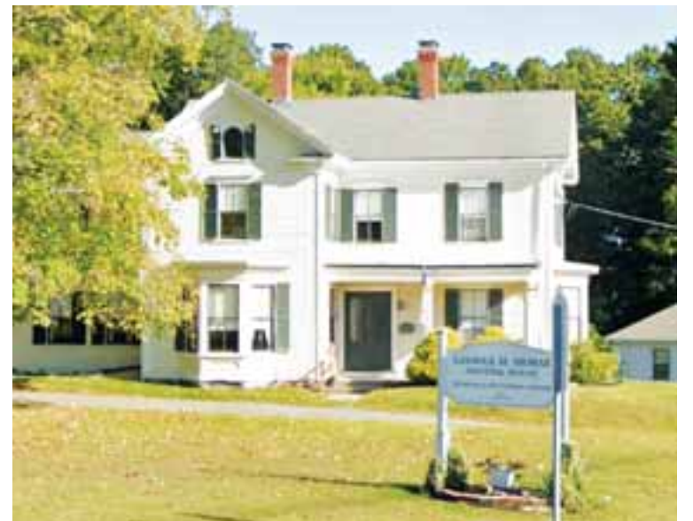
The Morse House as it currently stands on Washington Street.
